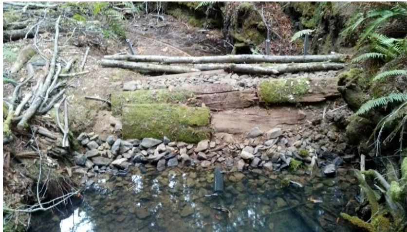
(Looking Downstream at the Dam)
