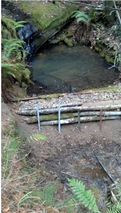
Photo 8 (Over Head view of Dam)
